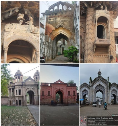
Figure 3 The Stucco work on some buildings of Lucknow
